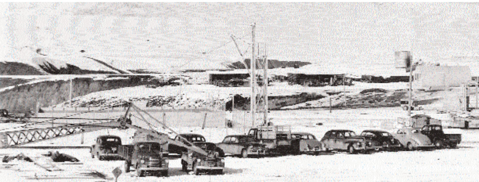
Jumping Pound Sulphur Plant, 1952.
