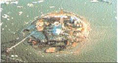
Issungnak, site of several wells drilled in shallow waters of the Beaufort Sea during the 1970s and '80s. The wells were drilled from "sacrificial beach islands" created by dredging gravel and sand from the ocean floor. Photo courtesy of Imperial Oi Limited.
