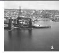
Sedco 135-F, the first offshore drilling vessel constructed in Canada, was commissioned in a dockside ceremony in Victoria in 1967. The semi-submersible platform cost \$10 million to construct and was capable of drilling to depths of 3,700 metres. Photo courtesy of Shell Canada Limited.
