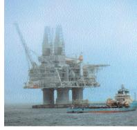
The Hibernia platform has a design capacity of 21,500 cubic metres to 23,850 cubic metres of oil per day. *Photo courtesy of Chevron Canada Resources-HMDC.*
