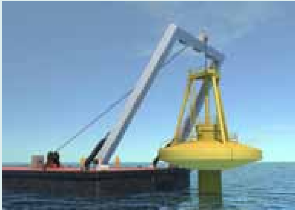
Figure 20 Device installation and O&M studies for the PowerBuoy point-absorber wave device
